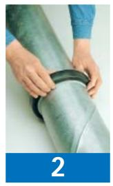
Align the connecting pipe's end with a clearance of 2-3 mm. Slide the rubber gasket over the joint.
