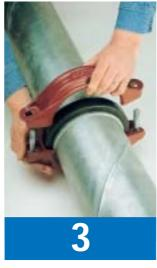
Fit the two halves of the coupling so that they enclose the gasket and the pipe ends.
