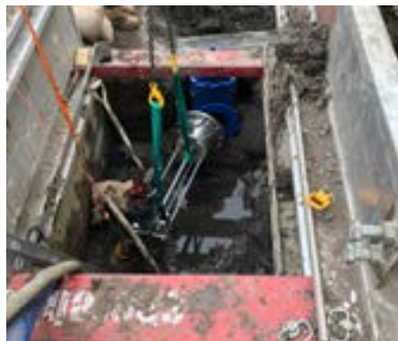
The existing main was underneath the water table, so continuous pumping was necessary to be able to conduct the weld and perform the hot tapping. The Plasson Large Bore Saddle was installed with minimal digging and lightweight equipment.
