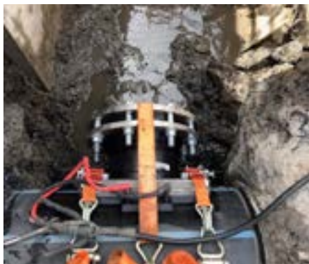
The existing main was underneath the water table, so continuous pumping was necessary to be able to conduct the weld and perform the hot tapping. The Plasson Large Bore Saddle was installed with minimal digging and lightweight equipment.
