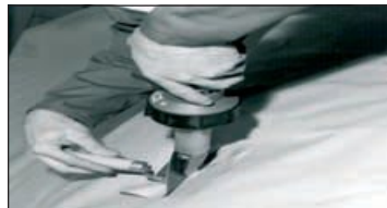
Hot-air welding of a patch seen from the
