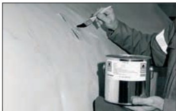
Application of adhesive.
