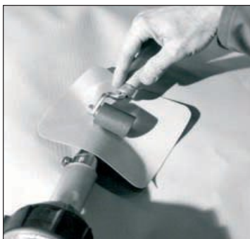
Hot-air welding of a patch and use of the pressure roller.
